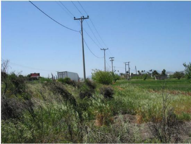
Figure 1. The location where the fire started, next to the National Road 1. Some burned shrubs are seen in the foreground. The electric power transformer suspected for causing the fire is visible at a distance in the middle of the photo (Xanthopoulos G. et al).
